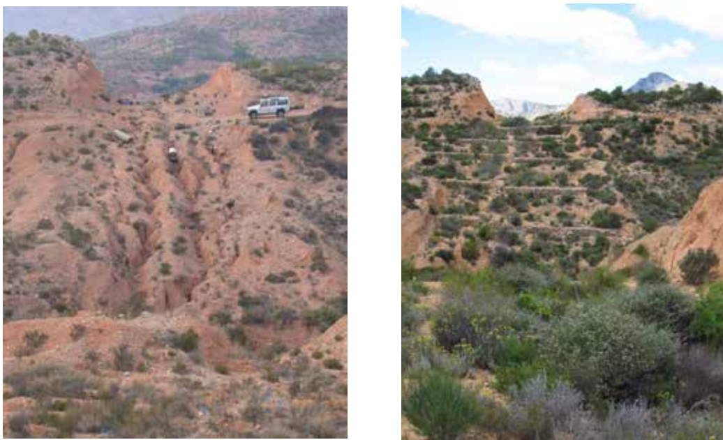
Figure 8. Degraded water pipe channel (left) and several years after the New restoration (right).
